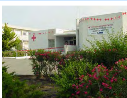
CRCS Central Offices, from where most of the help originates
